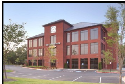
Mr. Smith uses the Managed Access Control solution at the Elizabeth Station building in Marietta, Ga.
